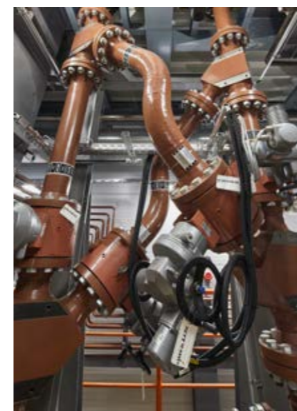
Delivery line cross connection
