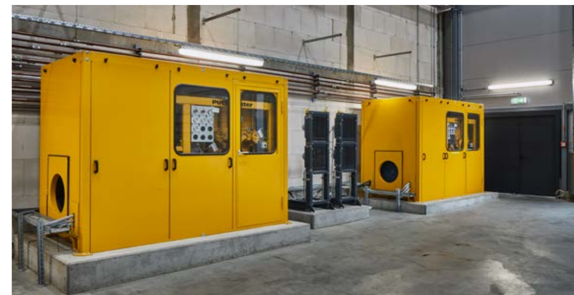
Hydraulic power packs with noise protection hood and external oil cooler
